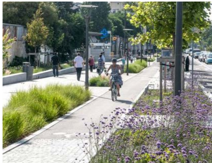
Figure 19: Swales feature within streetscape
